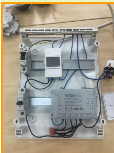
Electrical parts used in making the model in the IVVEC
